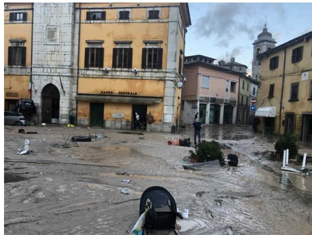
Figure 10: Flood damage in Cantiano , Italy, September 2022. Credit: Mayor of Cantiano Alessandro Piccini
