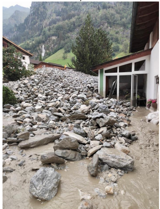
Figure 8: Flood and mudslide damage in South Tyrol region, Italy, 05 August 2022.
