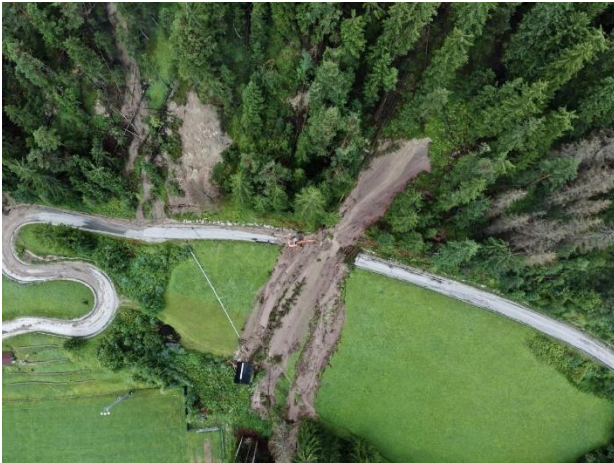
Figure 6: Heavy rain triggered flood and landslides which cut roads in San Martino in Badia, Italy, 05 August 2022.
