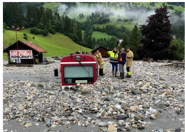
Figure 5: The Krimml station, track and a train of the Pinzgauer local railway in Wald im Pinzgau were completely buried. Photo Wald Municipality
