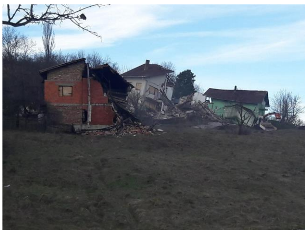
Figure 7. Landslide damage in Hrvatskoj Kostajnici, Sisak-Moslavina County, Croatia, 13 March 2018. Credit: National Protection and Rescue Directorate Croatia (DUZS)
