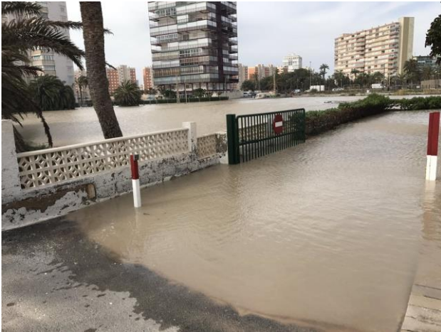
Figure 5. Floods in Playa de San Juan, Alicante, March 2017. Photo: Office of the Mayor of Alicante
