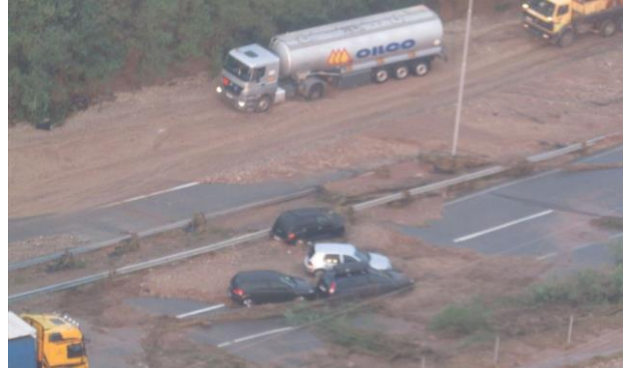
Flooding caused major damage to the road network. Photo courtesy of Macedonia Ministry of Interior.
